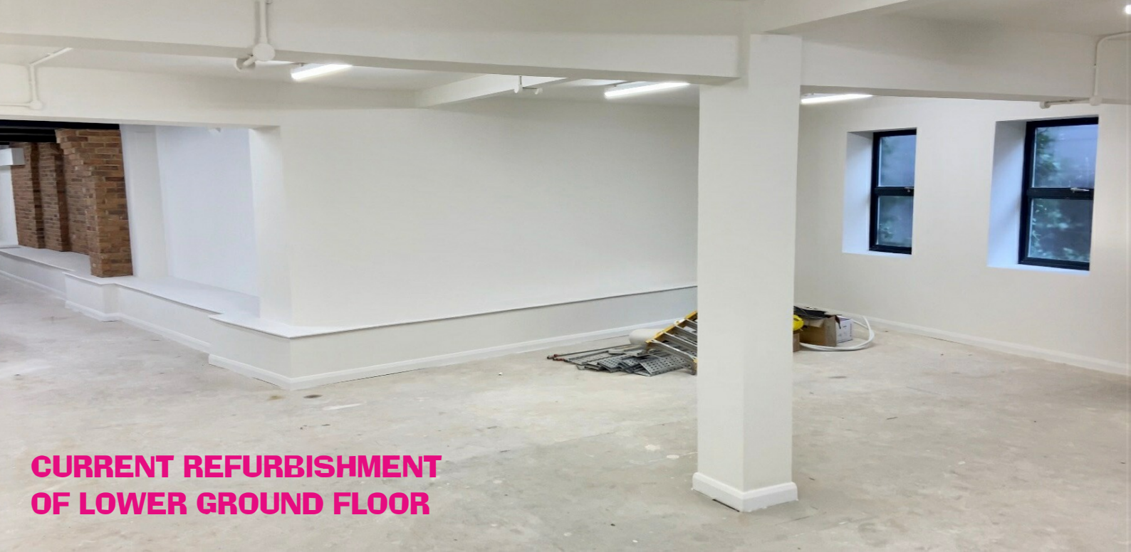
CURRENT REFURBISHMENT OF LOWER GROUND FLOOR
