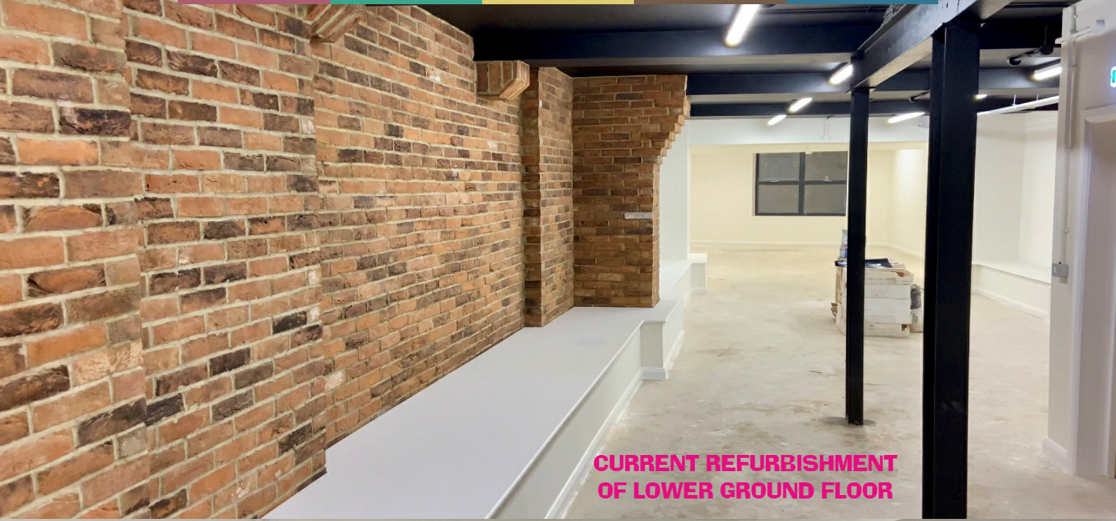
CURRENT REFURBISHMENT OF LOWER GROUND FLOOR
